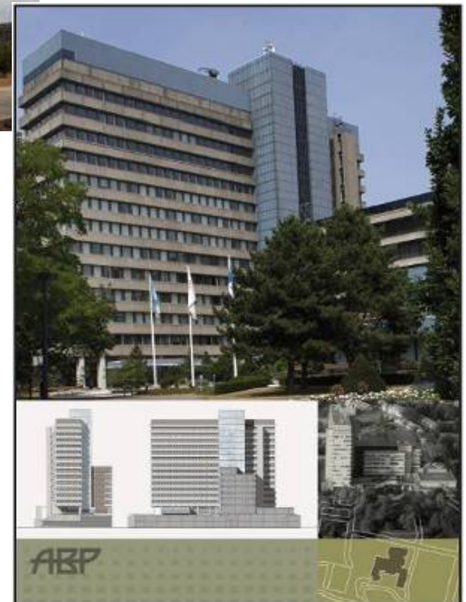
ABP building (retrofitting)
