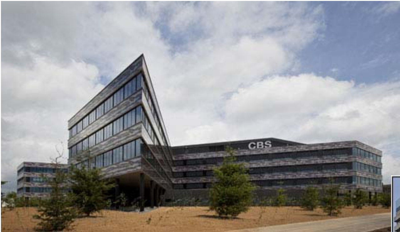
CBS building (new office)
